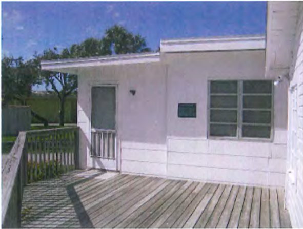
The annex at 161 Bay Road
