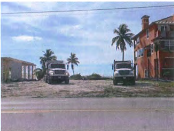
3120 ESTERO BOULEVARD (Comp Plan historic structure #8LL01546 demolished in 2013)
