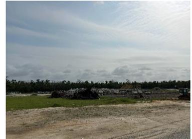
The concrete will be crushed and along with the dirt used as fill for the new softball field, as the area needs to be raised about three feet to prevent future flooding. Our staff take precautions daily to keep the children clear of the debris and we have created a new entrance for the hauler trucks to enter on the opposite side of Bay Oaks Park. Safety is our number one priority, which is why a fence will be installed soon near the playground to prevent anyone from getting too close.
